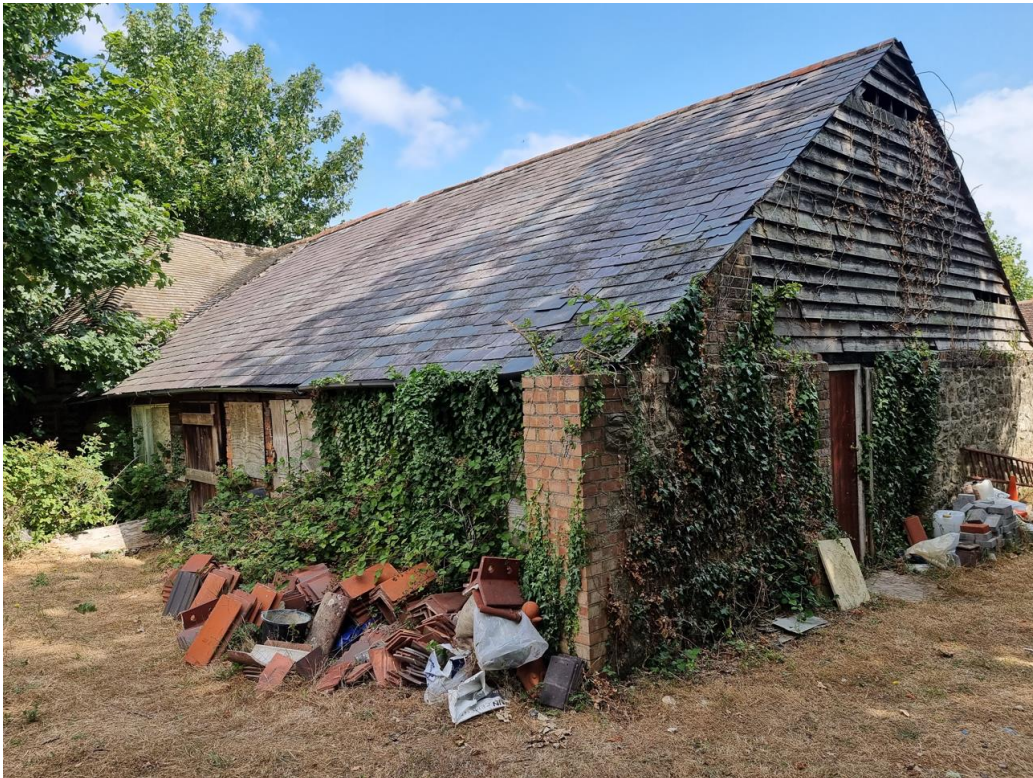
Fig 4. Rear (east) elevation. Cart store (in foreground) with Granary building attached.
